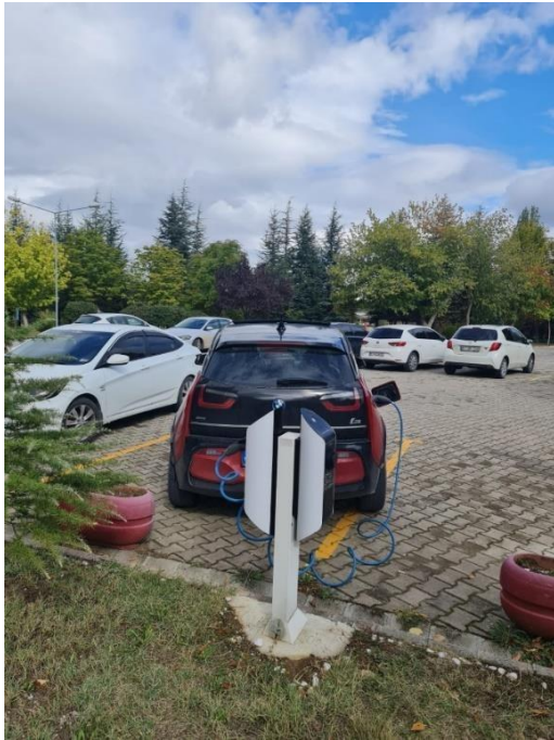
dual AC charging point and sample electrical vehicles 3
